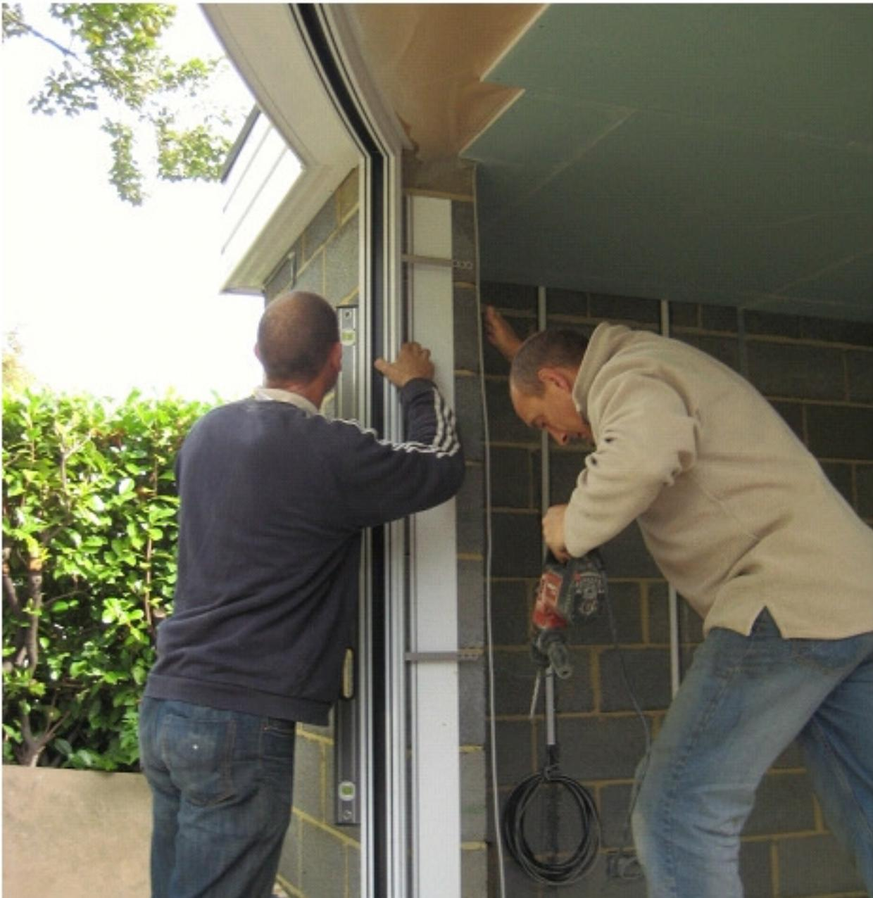
4) Get ready to insert the doors onto the track. Identify the doors and decide which to insert first so as to have the most comfortable access and hold on the doors, as you insert them.
