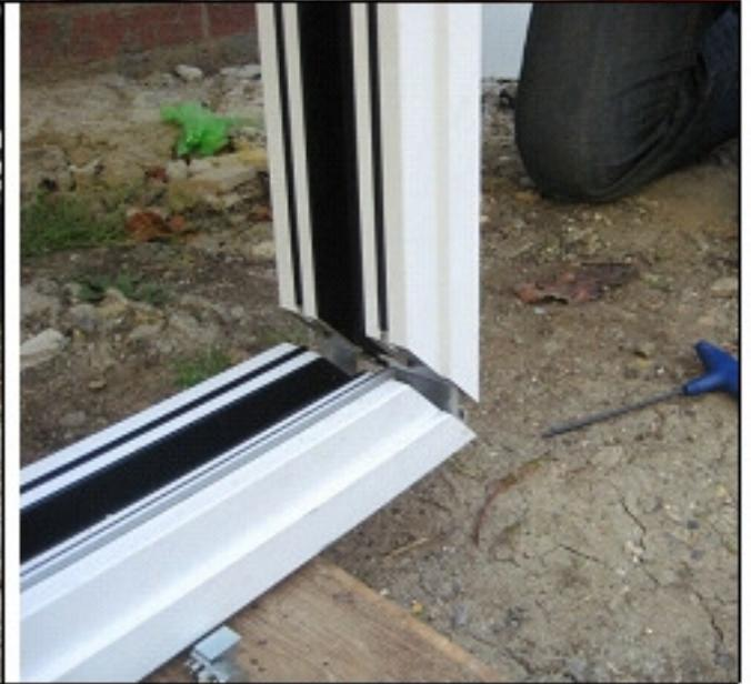
You may need to support the top frame with temporary supports so it does not sag until it is installed.
